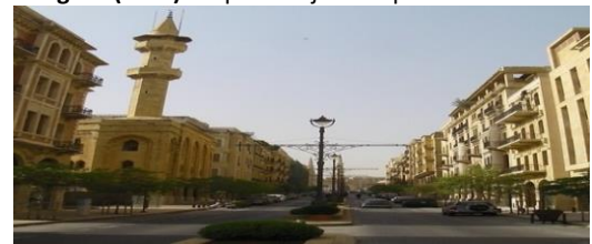
Figure (12-B): Shows Rue Foch after the completion of conservation works (32) .
