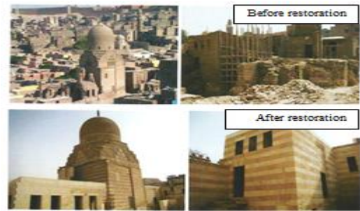
Figure (15-B): Tarbay Al-Sharief Complex before and after restoration (25).
